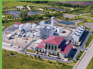
Faribault Energy Park 300 MW, Natural Gas/Steam
