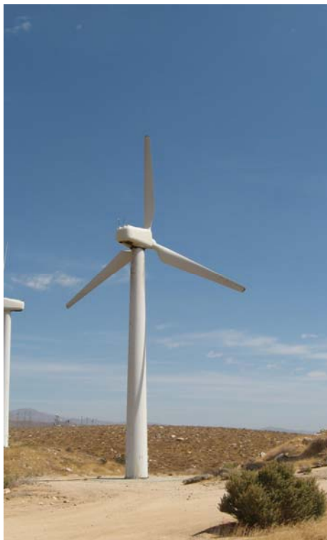
An example of a 160 KW wind turbine
